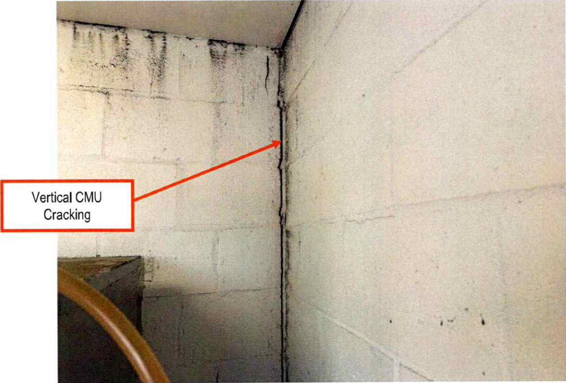
Figure 6: Building 3 Meter Room
