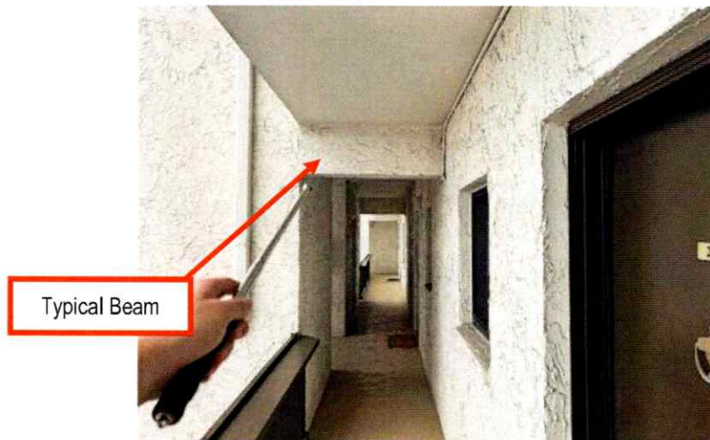
Figure 3: North Elevation Walkway
